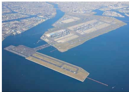
The newly opened fourth runway. (C) Haneda Airport Expansion Project JV
