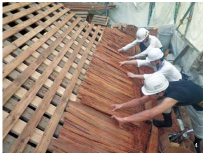
1. Hiwada buki roof of a building at Kumano Hongu Taisha Shrine (Photo: PIXTA) 2. A motokawashi climbs a tree over 10m tall to collect the outer bark. 3. A special knife is used to shape the bark. 4. Cypress bark soaked in water is laid out side by side. 5. Structures are roofed with great precision using different layering techniques on different areas of the roof. (Photos 2–5: National Society for the Preservation of Shrine and Temple Roofing Techniques)
