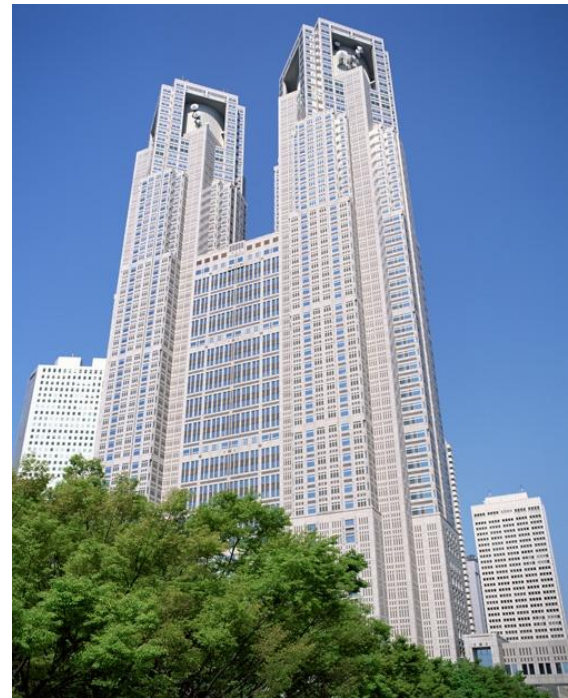
Tokyo Metropolitan Government Buildings
