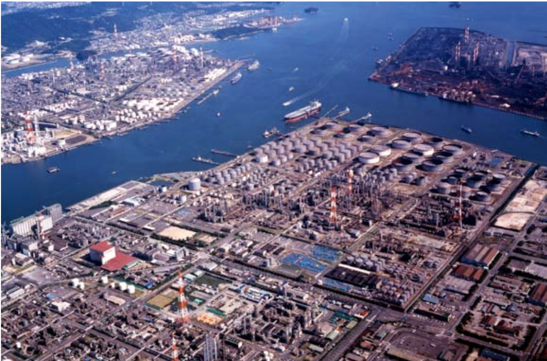
A petrochemical complex © Nippon Oil Corporation
