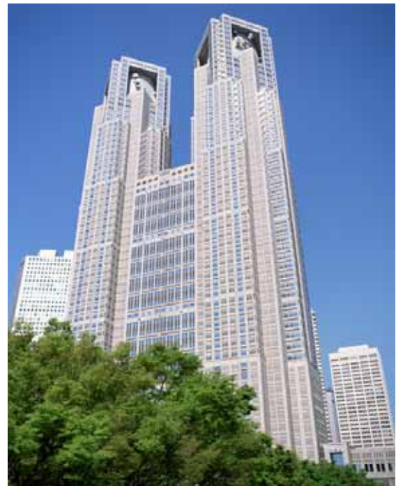
Tokyo Metropolitan Government Buildings
