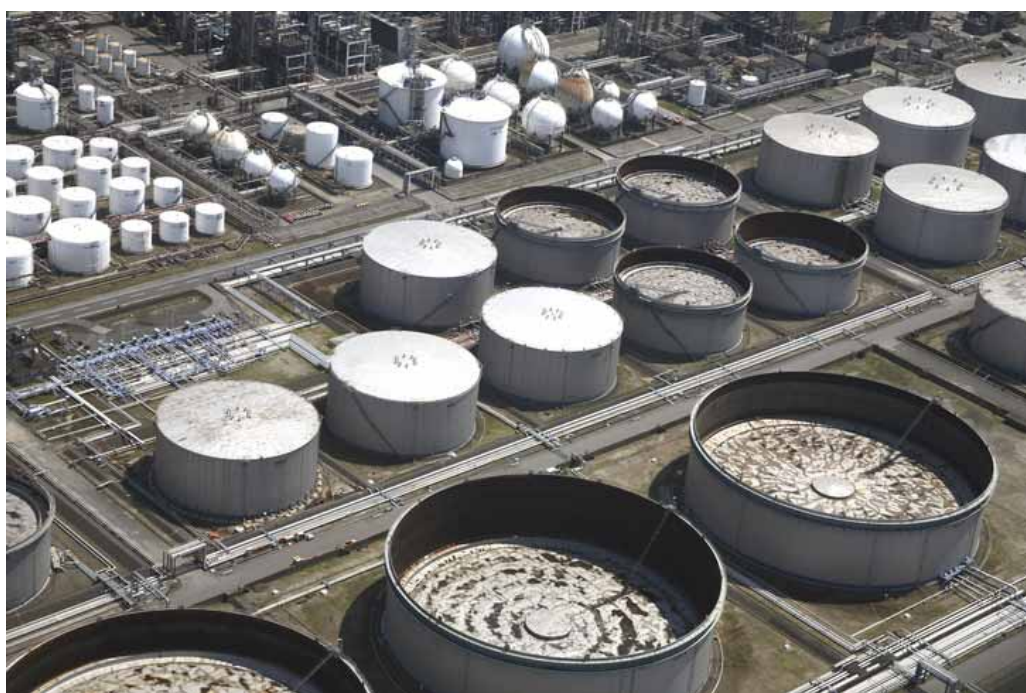
A petrochemical complex (Photo courtesy of AFLO)
